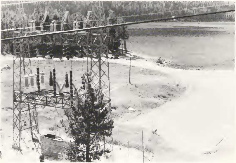
Fig. 1 Adams tunnel gate house site with photographer facing south toward Grand Lake. Intake structure and conduits to gate house are buried under paved roadway and parking area at the right side of the picture. Photo by G.F. Price.
